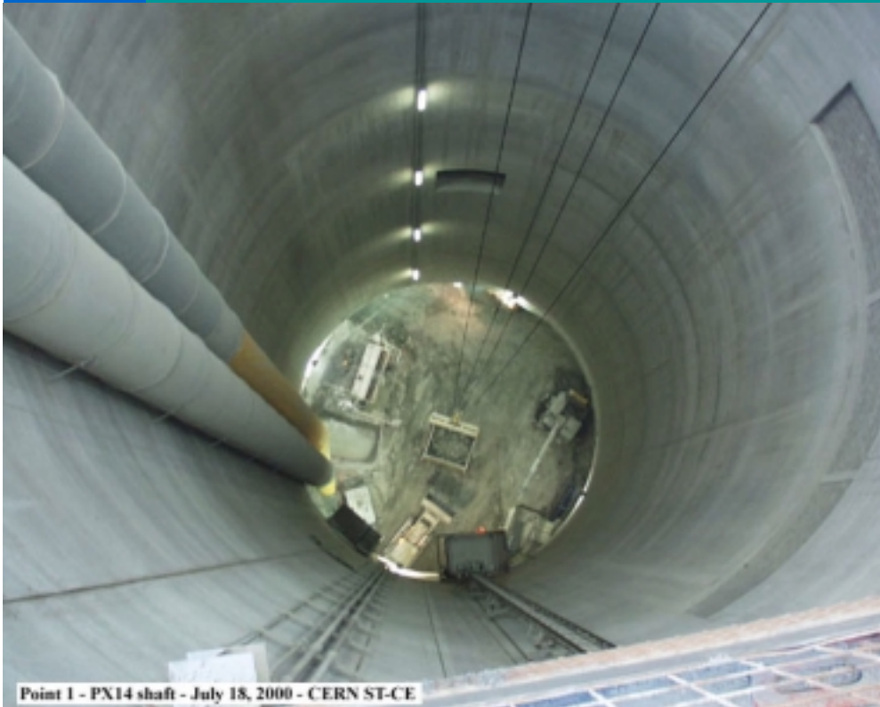
Point 1 - PX14 shaft - July 18, 2000 - CERN ST-CE
