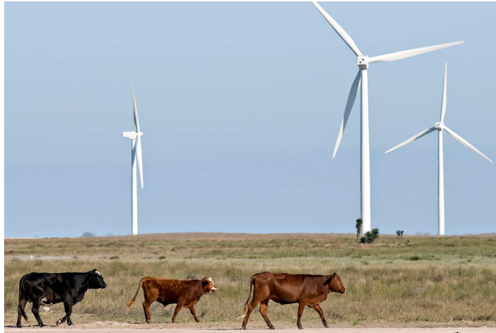
Figure 4: Windmills on a Texas wind farm along the Gulf coast. Wind strikes windmill blades attached to the shaft of an electric generator inside the horizontal structure (“nacelle”) atop a tower. The shaft then rotates so that the wind now becomes the hand of Fig. 2.
