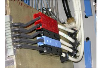
**Low voltage cables and connectors**
