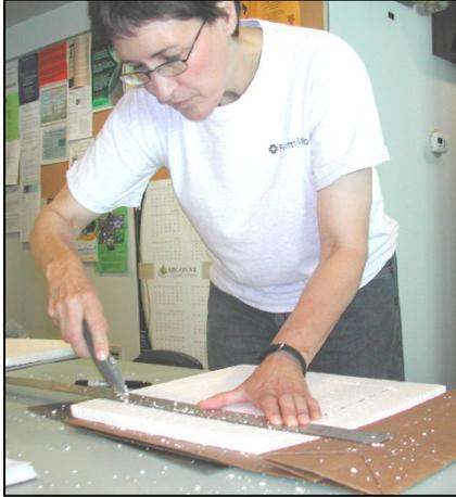
**B) Cut the foam insulation to size.**
