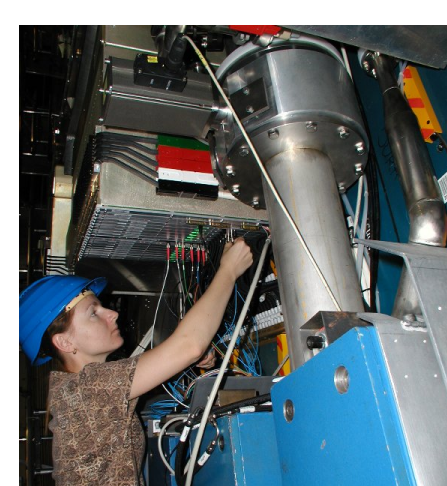
SMU physicist is installing the optical link to the FEBs in the front-end crate
