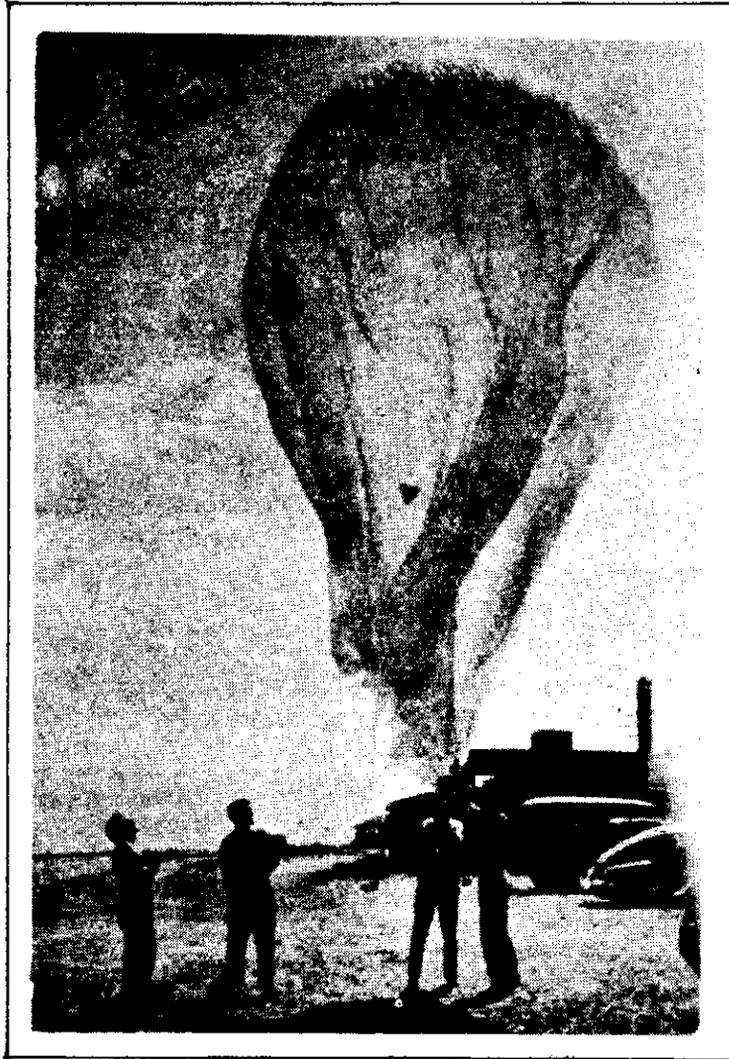
Figure 12: Neoprene balloon encased in a nylon shroud
